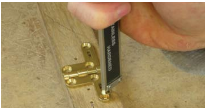
Use a Vernier gauge to measure the depth of the screw
