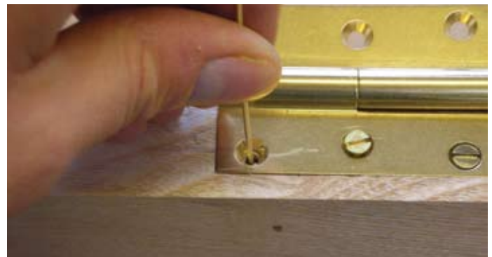
Insertion of a small piece of wood will move a screw over slightly to one side
