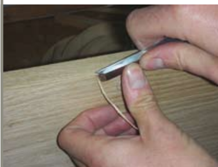
Trimming back with a chisel
